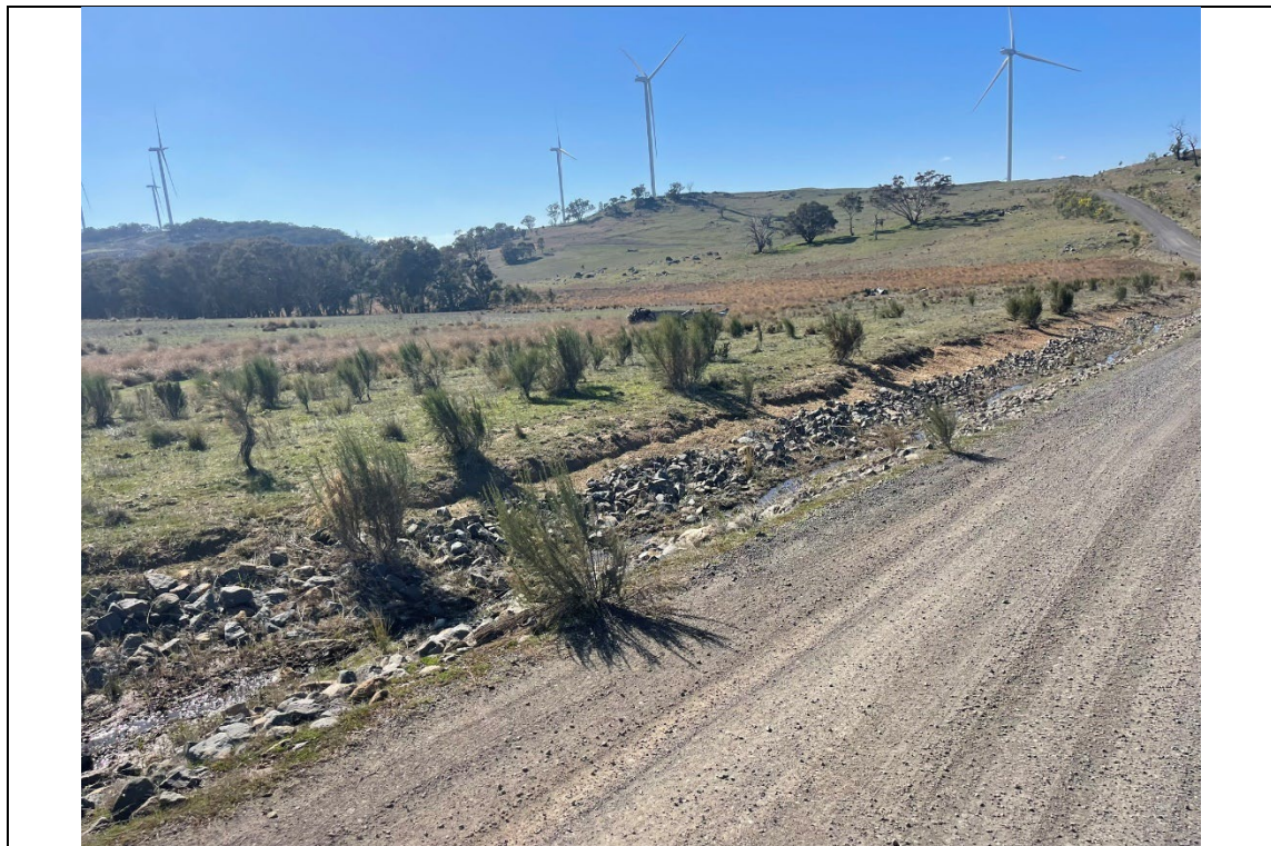
Photo 16 Rock-lined swale drains.
