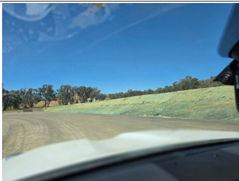
Ongoing rehabilitation works. Soil binder has been sprayed on the embankments to control dust emissions.
