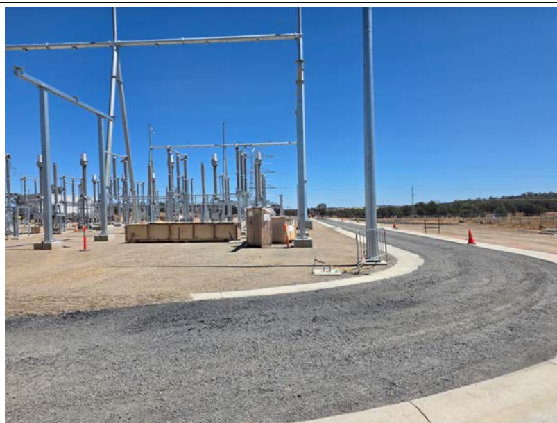
Transgrid Switching Station: Permanent road and kerb works ongoing around the Areas 1 and 2.
