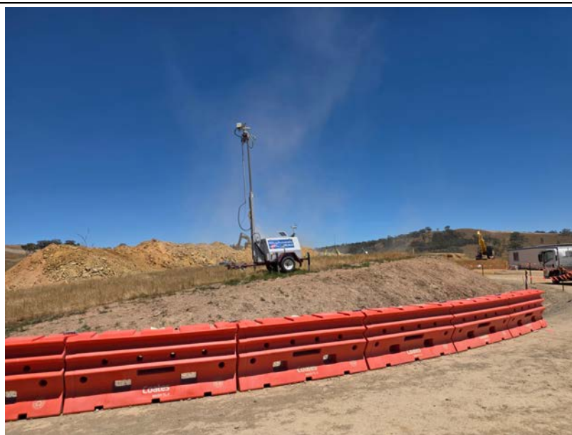
Transgrid Substation: Visible dust observed to be generated from crushing activities on site. A non-compliance has been raised against CoA B16 due to lack of dust suppression controls during the crushing activity.
