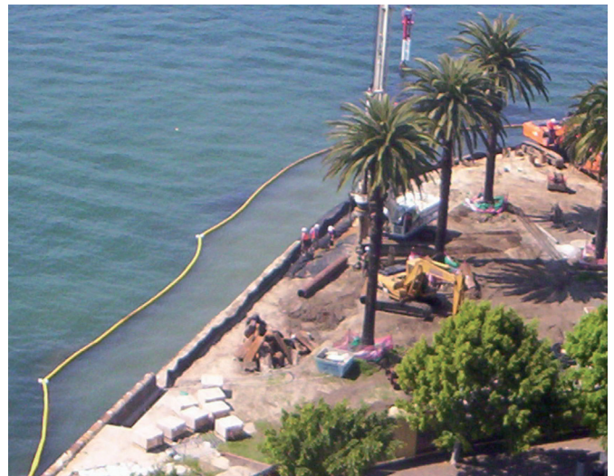
▲ Boom contains spill near bank. Note the boom is anchored into position.
