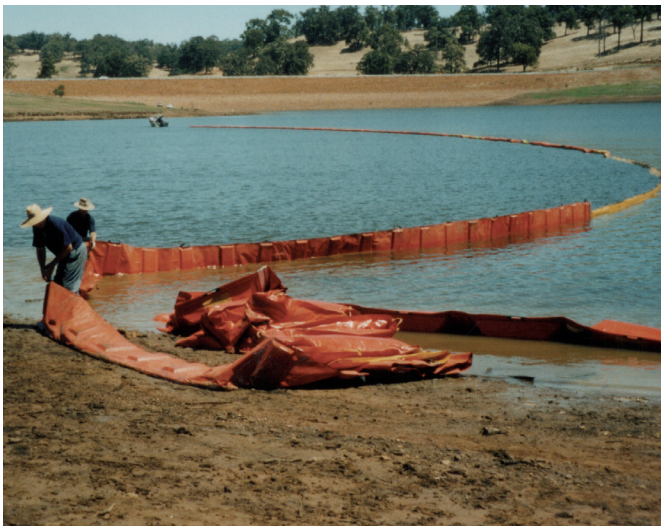
▲ The boat heads into the wind to enable the deployment of the boom
