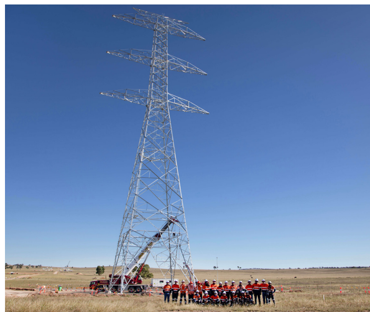
Australia’s first REZ transmission tower completed. Credit: EnergyCo
