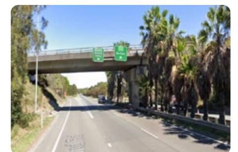
Below: Tarro Interchange overpass - 6.2m clearance.
