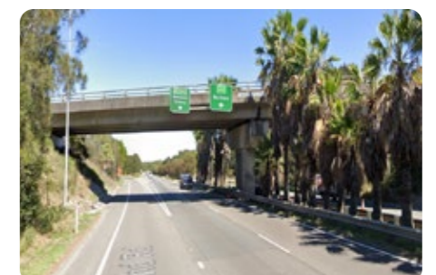
Below: Tarro Interchange overpass - 6.2m clearance.
