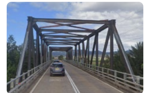
Above: Denman Bridge - 5.8m clearance.
