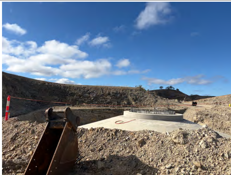
WTG foundation works ongoing
