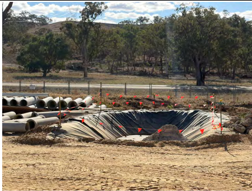
Transgrid Substation: Concrete washout area observed to be satisfactory
