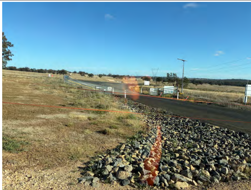
Rock dams and asphalt installed around site entrance
