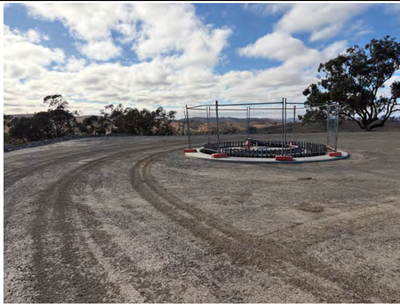
WTG foundation works ongoing
