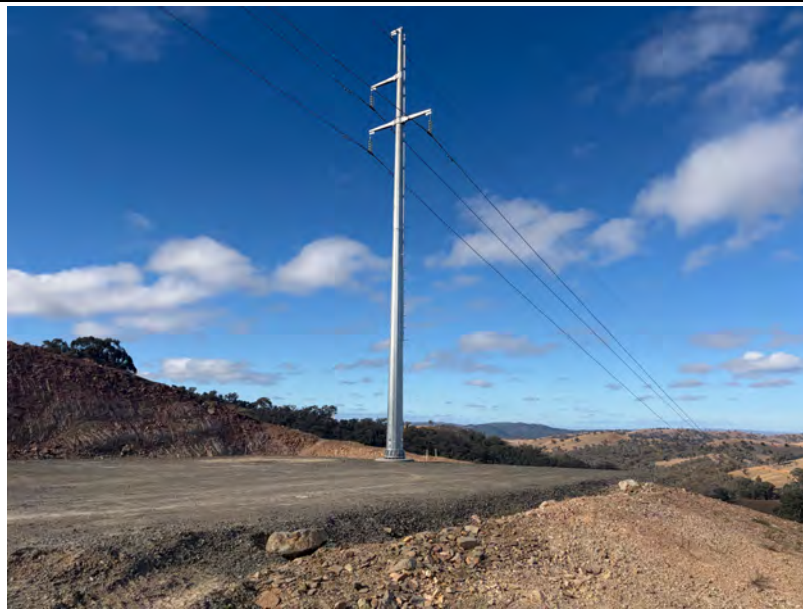
33kV overhead powerline works
