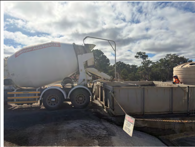
Concrete agi washout area operations ongoing at the batching plant
