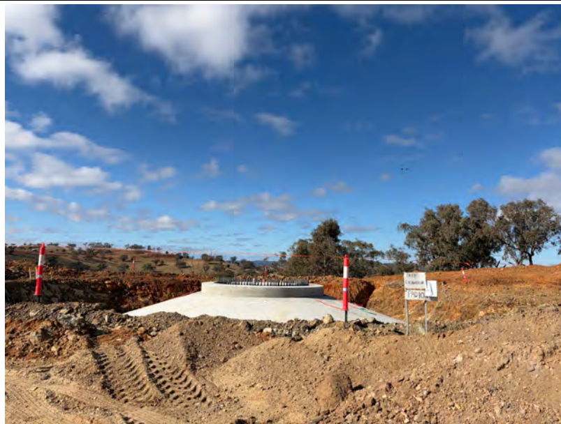
WTG foundation works ongoing at PAD 102
