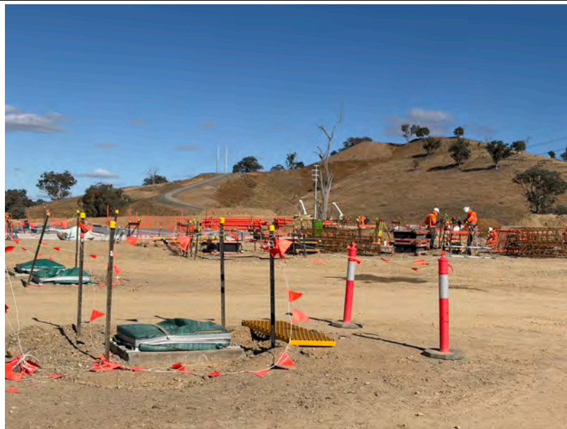
Transgrid Substation: Drainage installed and protected
