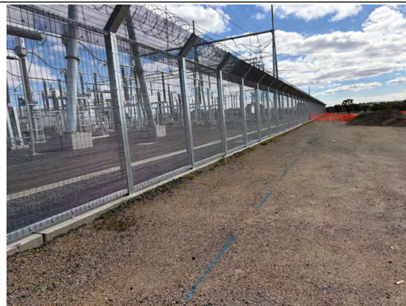
Transgrid Switching Station: Landscaping works being planned
