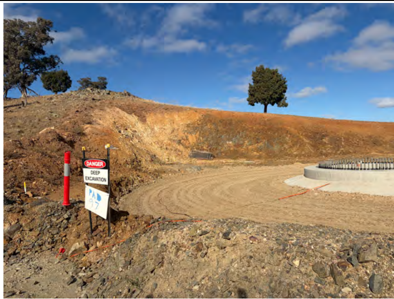
WTG foundation backfilling and compaction ongoing at PAD 98
