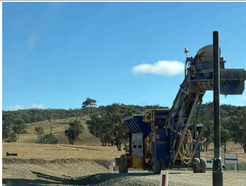
Crusher plant being relocated
