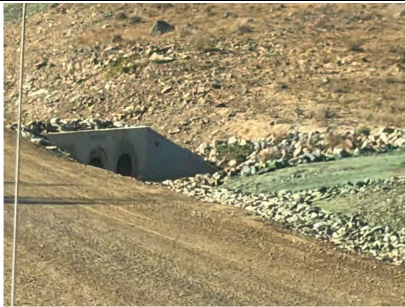
Culverts installed and surrounding areas stabilised with polymer and rock checks
