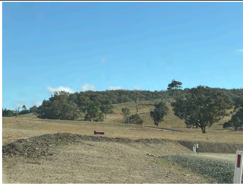
Mulch berms in place
