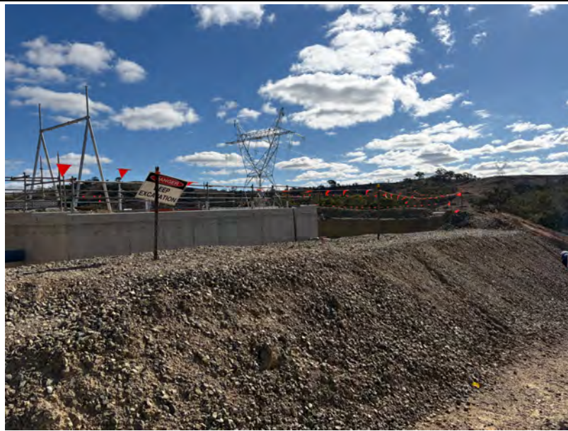
Transgrid Substation: Oil/water separator tanks installed
