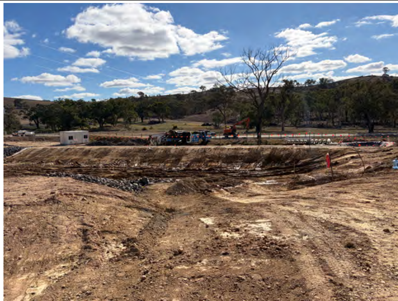
Transgrid Substation: Sediment basin maintenance ongoing
