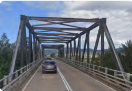
Above: Denman Bridge - 5.8m clearance.
