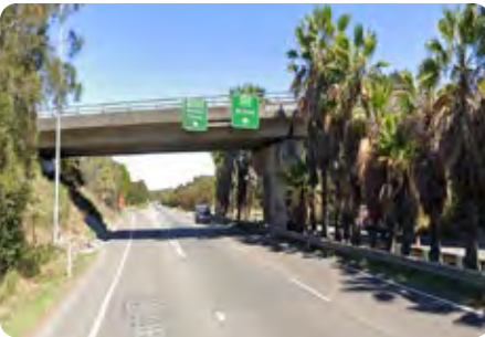
Below: Tarro Interchange overpass - 6.2m clearance.
