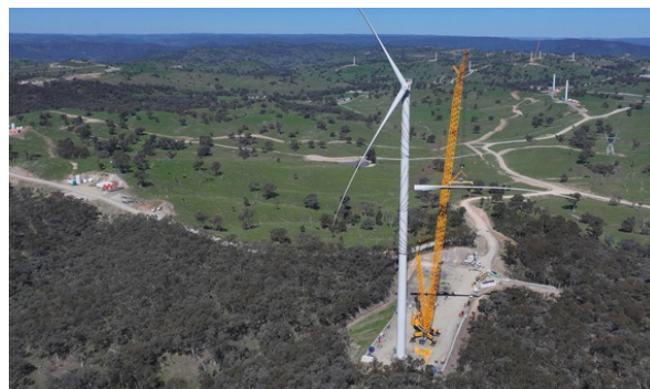
The third blade being lifted up by a 1,000 tonne crane
