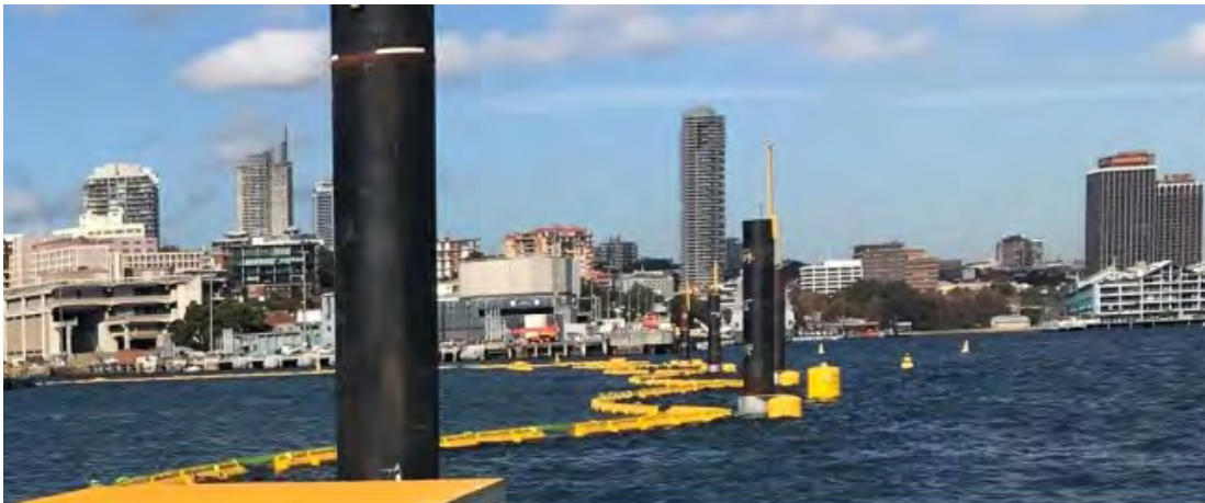
Figure 10.1 Example of similar installations
