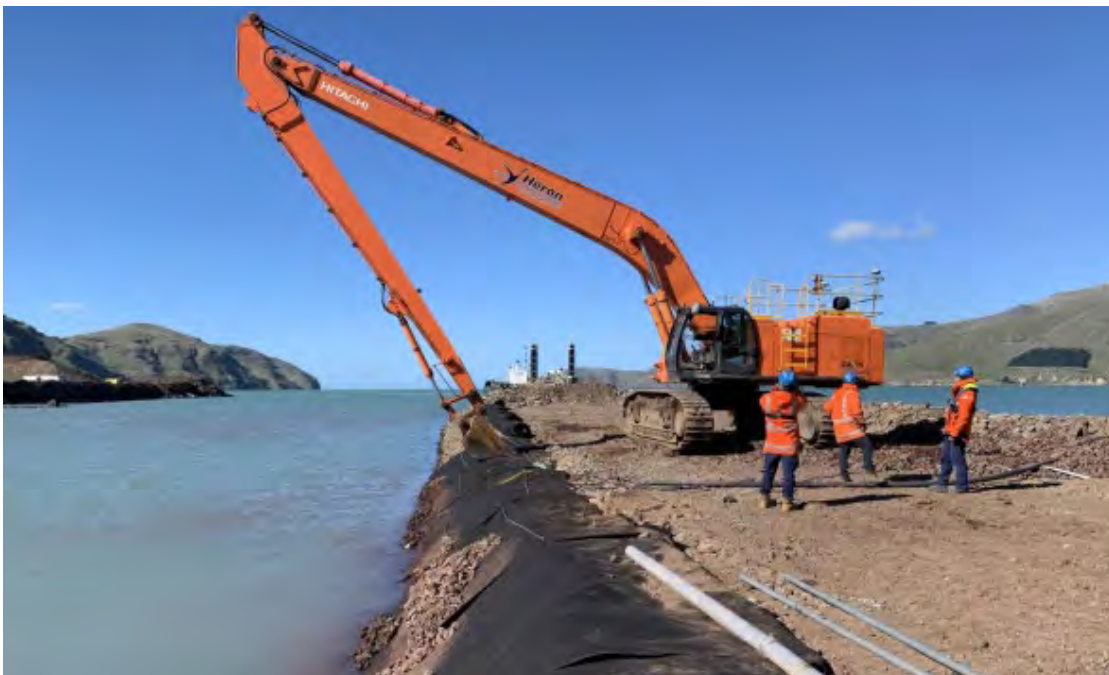
Figure 10.8 Longreach assisting in geotextile installation
