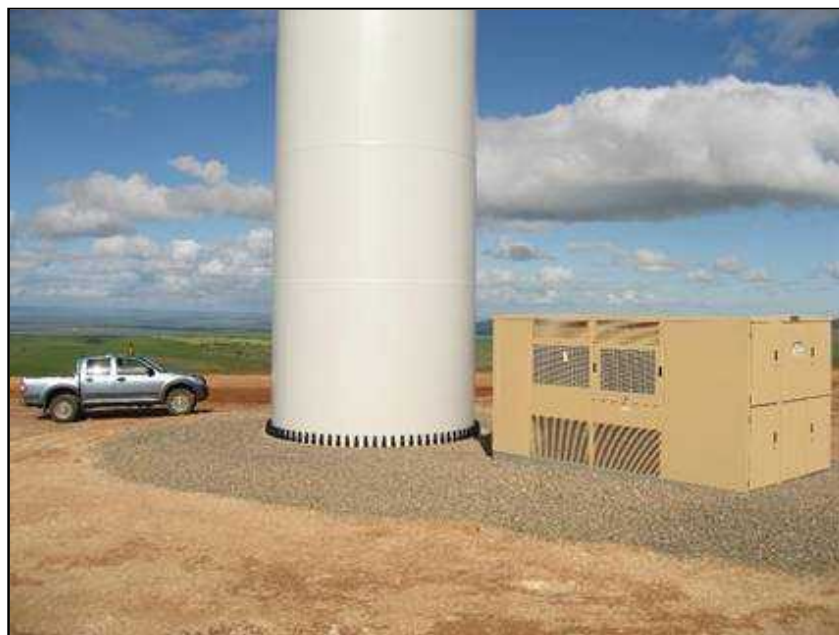
Image 3.5 Transformer adjacent to wind turbine
