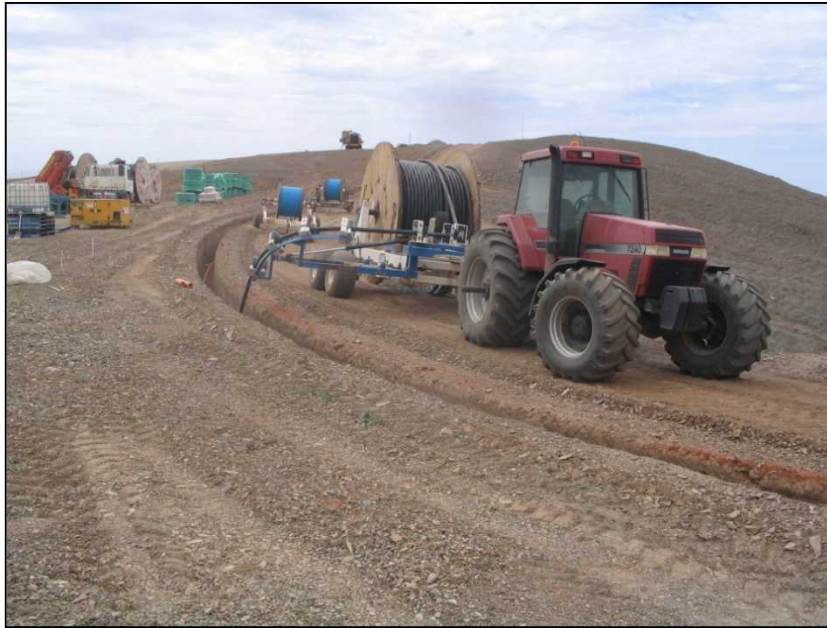
Image 3.7 Laying underground electrical cable within road network
