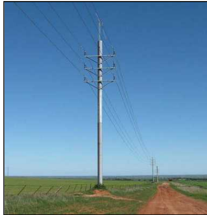
Image 3.6 Double-circuit overhead 33 kV power line
